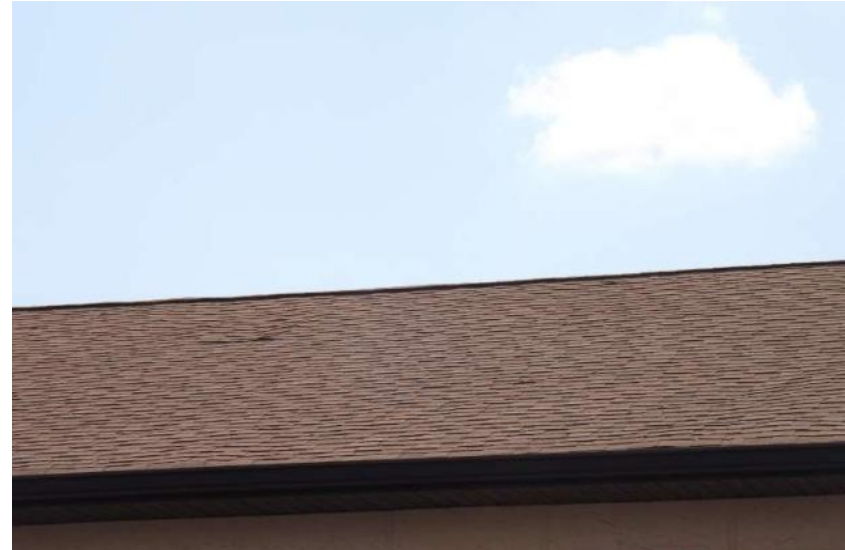
Asphalt/Fiberglass Shingle Roof Covering
