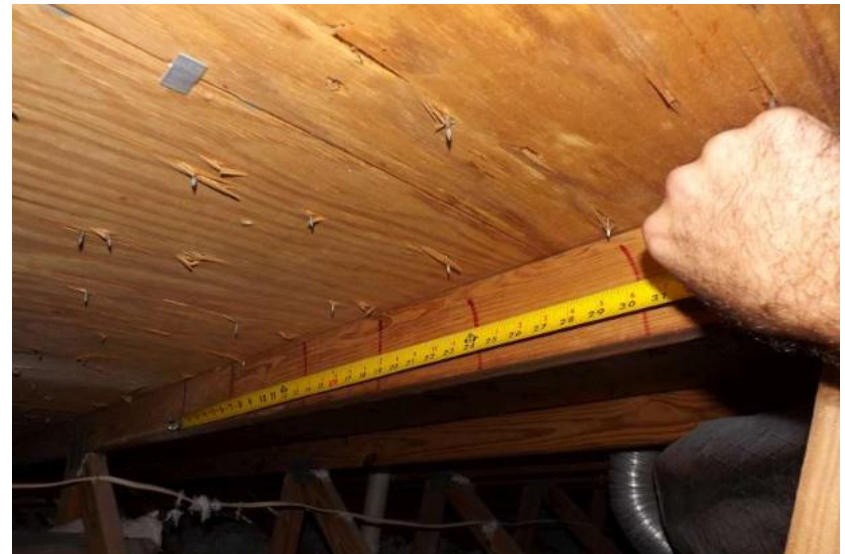
8d Nails Spaced 6" in the Field
