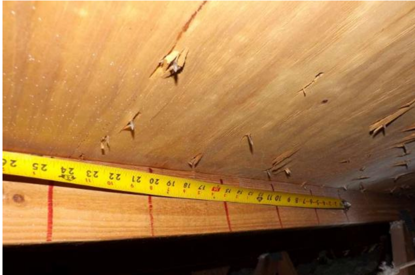
8d Nails Spaced 6" Along the Edge
